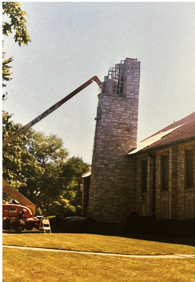
The bell tower being removed in September of 2002.
