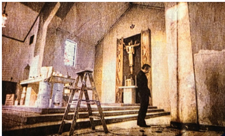
Mmgr. Zollinger inspects the damage from the attempted arson.
