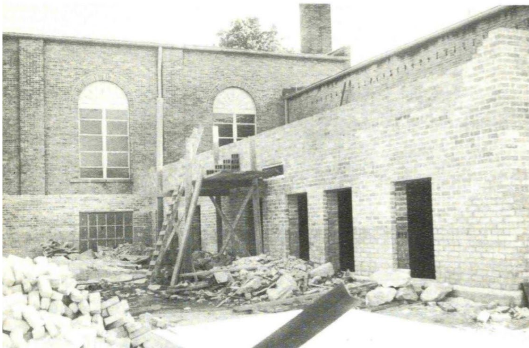
Rebuilding the school after the fire in 1940.
