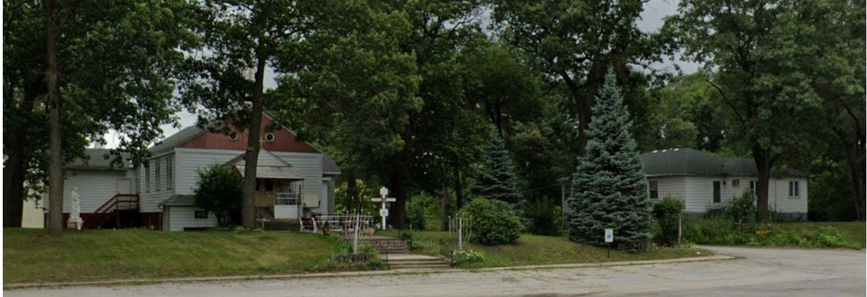
St. Ann Roman Catholic Church in the Black Oak neighborhood of Gary, Indiana. To the right of the church building is the parish rectory. After the school closed, the school building and convent were demolished, leaving just the rectory and church.
